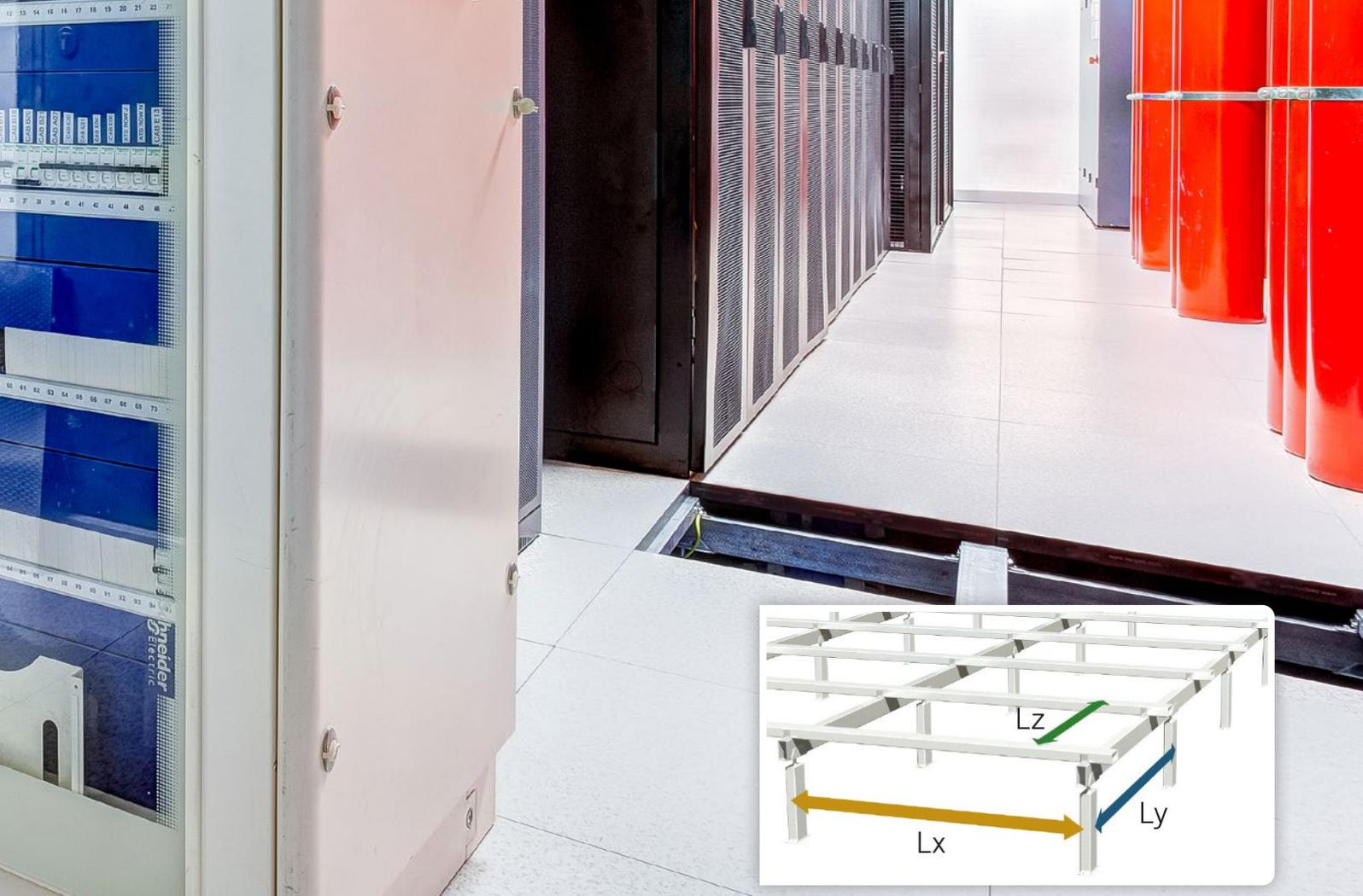
The distance between primary beam sections ( $L_x$ ) and pedestals ( $L_y$ ) are the factors that control the design load.
